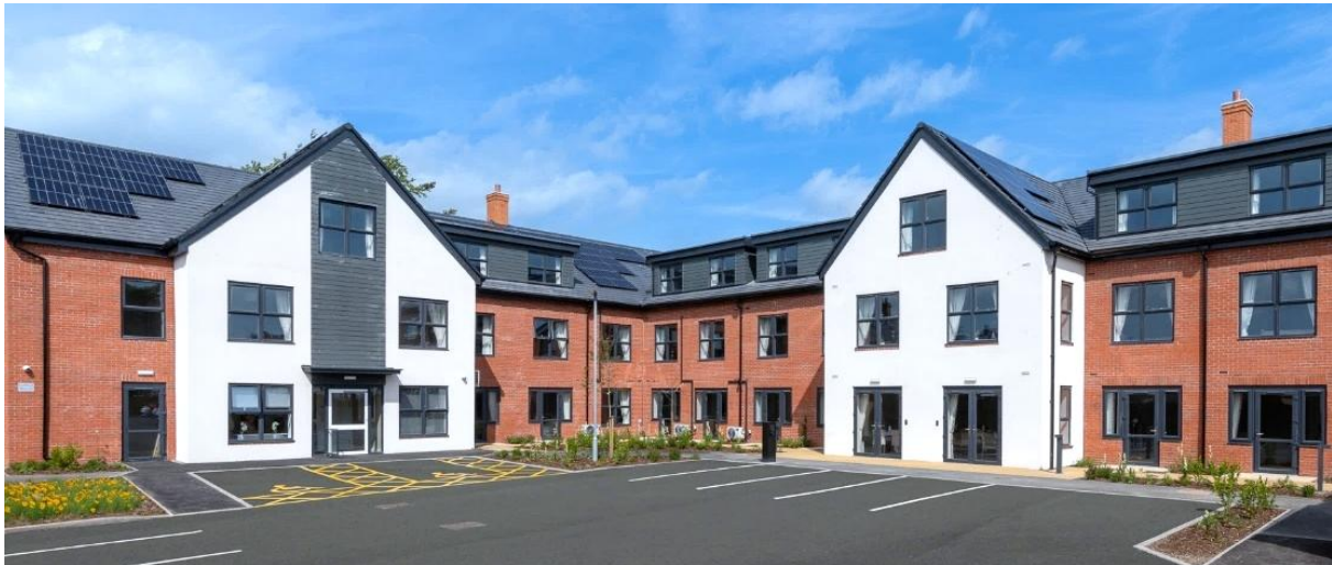
Beechwood Care Centre – Bridlington
