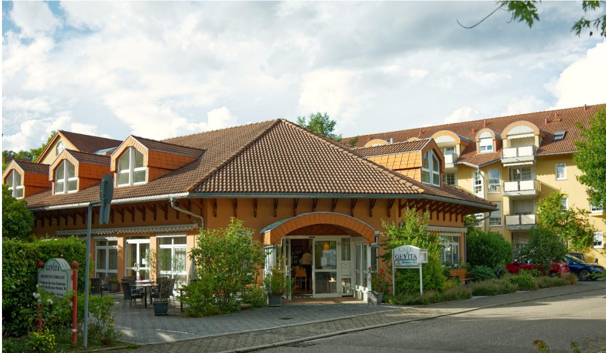
Gevita Residenz – care campus in Lörrach (DE)
