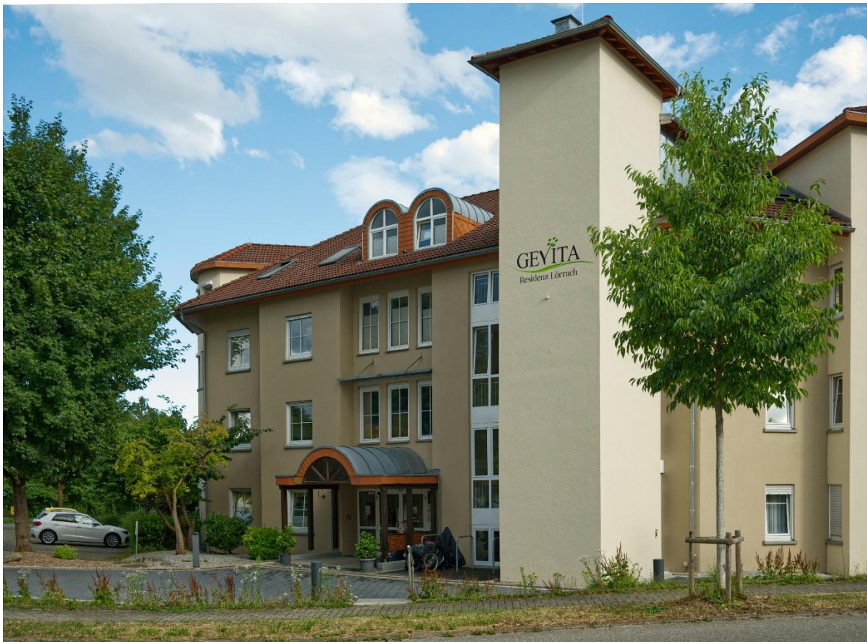
Gevita Residenz – care campus in Lörrach (DE)
