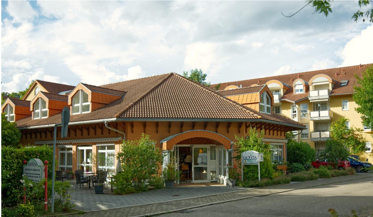
Gevita Residenz –Pflegecampus in Lörrach (DE)
