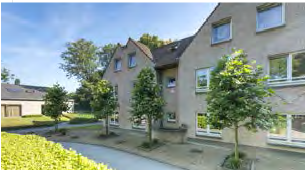
Helianthus Senior housing - Melle (Belgium)
