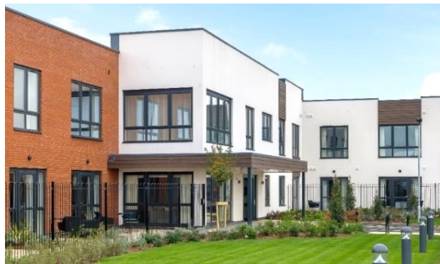
Chartwell Manor in Aylesbury, let to MMCG Care home completed in September 2022
