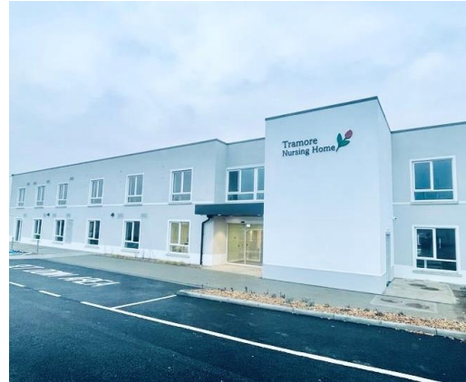
Tramore Nursing Home – Tramore (IE)
