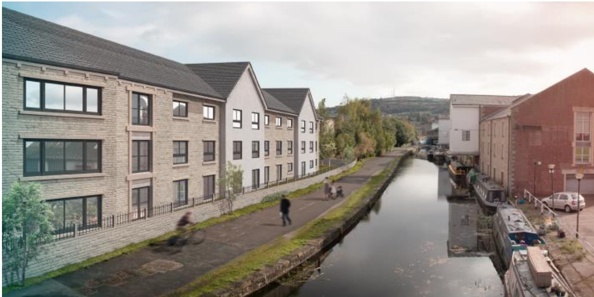
ShIPLEY Canal Works (impressie) – Shipley
