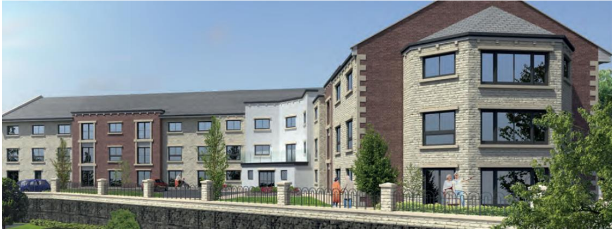
Shipley Canal Works (impressie) – Shipley
